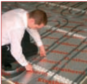
Below floor slab.
