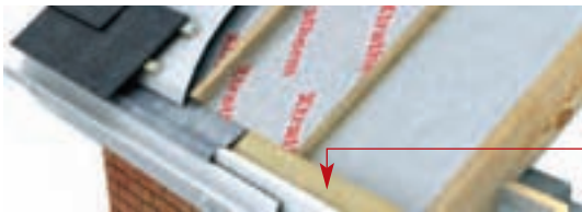
A timber stop rail is fixed to the bottom of the rafters
